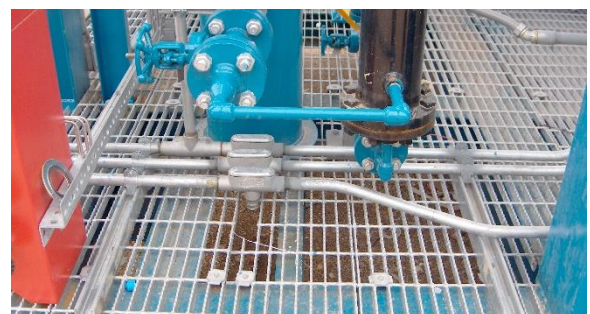
Figure 2. Electrical raceway installation. Grate was cut to provide enough space for drain fitting.
