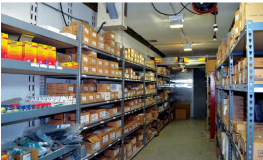
Figure 7. An example of a jobsite storage trailer for an electrical contractor.
